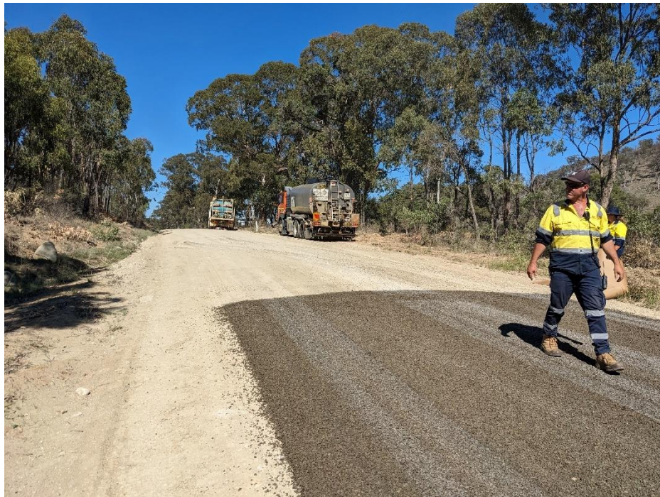
Image 1: Bitumen sealing Tent Hill Road
