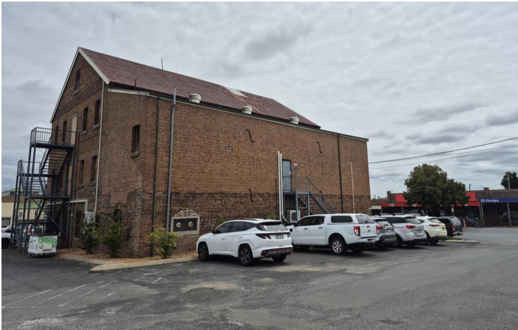
Figure 13 - Facing North East from central within car park
