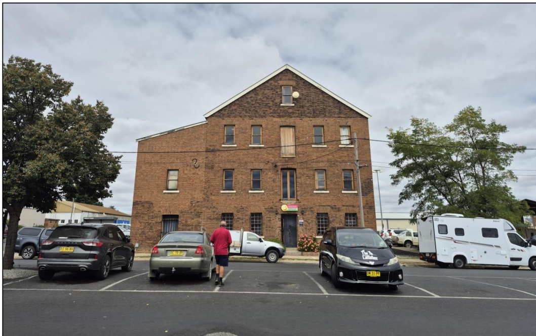
Figure 6 – Facing South from Bourke Street, showing front elevation of 177-179 Bourke Street
