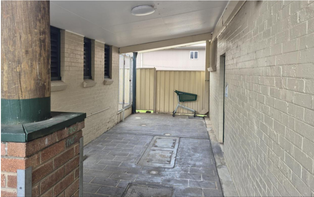
Figure 11 - Showing public amenities between buildings at 217 Grey Street
