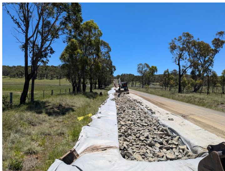
Images: Rehabilitation Works
