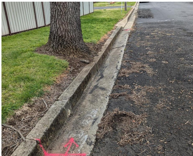
Image: Damaged kerb and guttering
