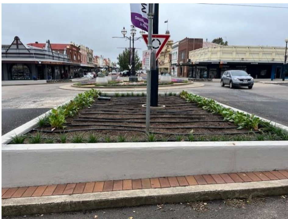
Image 5: Laying of watering system
