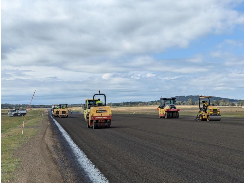
Image 1: Rolling bitumen
