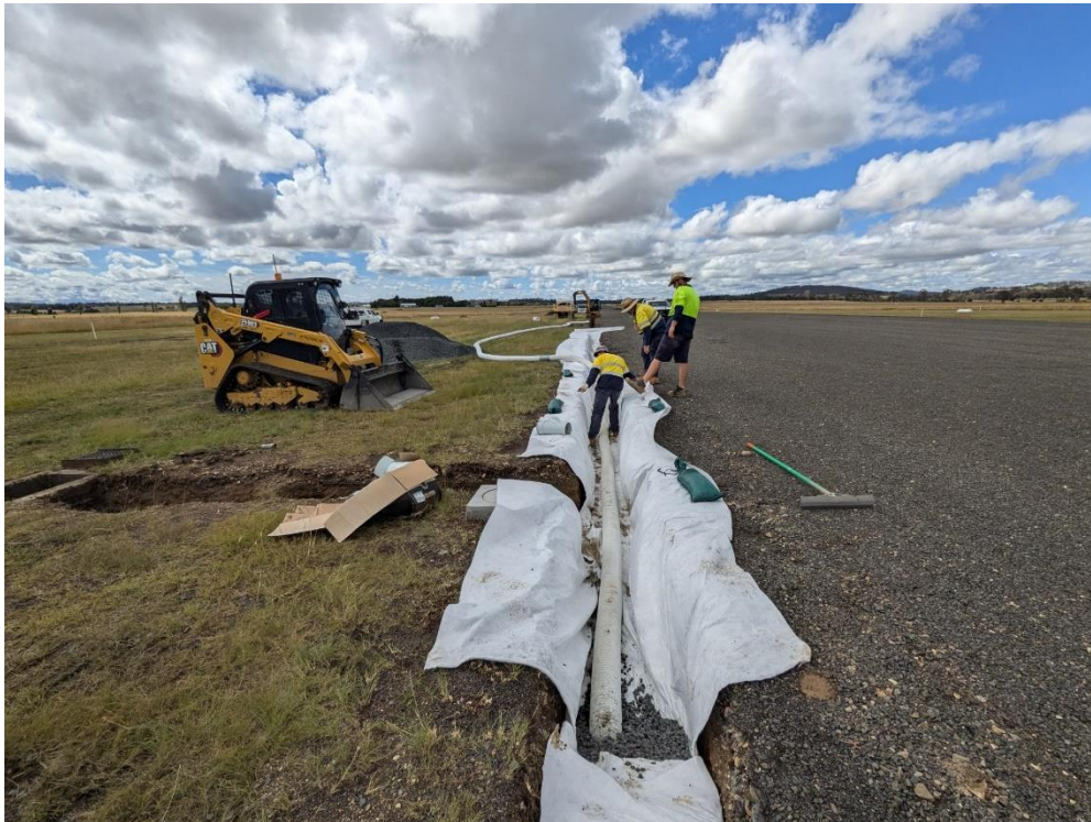
Subsoil drainage installation on Runway 14/32
