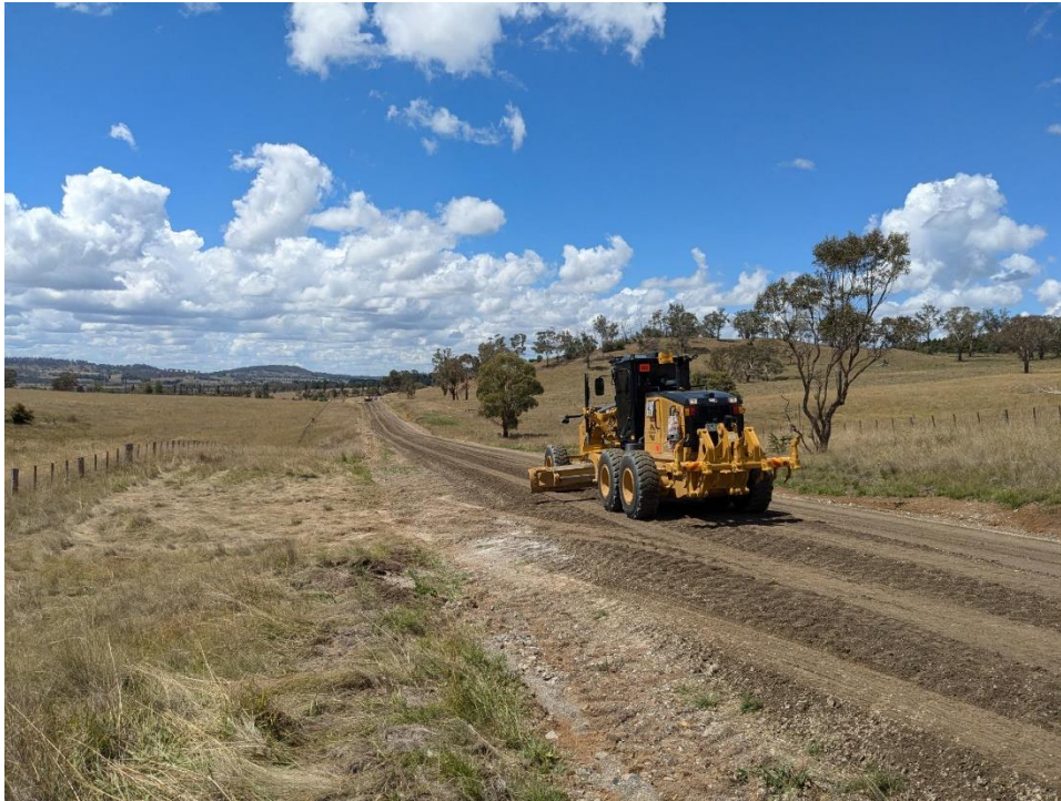
Stabilisation works on Haymarket Road
