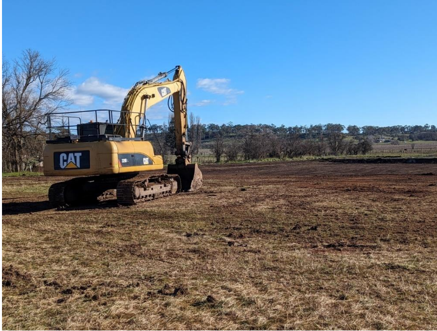
Image 2: Dumaresq Street subdivision earthworks
