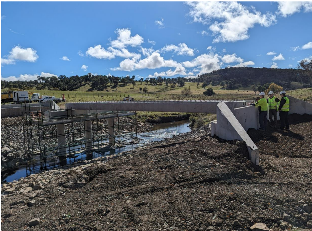
Image 1: Mt Mitchell Rd bridge
