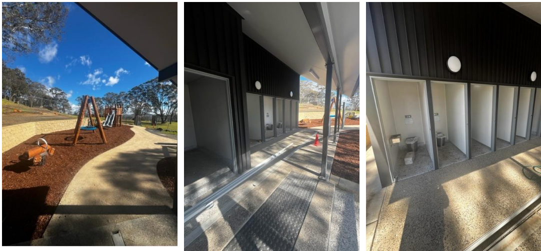
Image 4: Centennial Parklands Project – Construction
