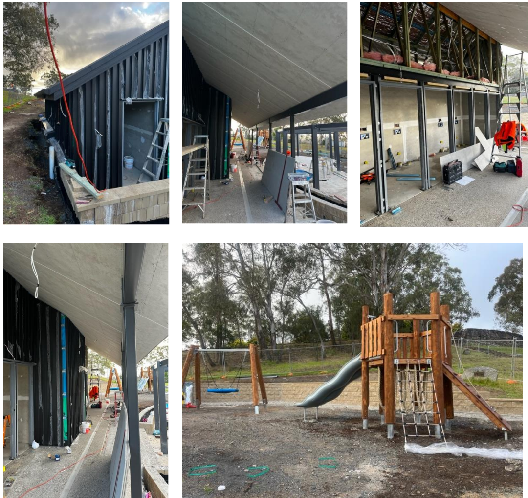
Image 4: Centennial Parklands Project – Construction
