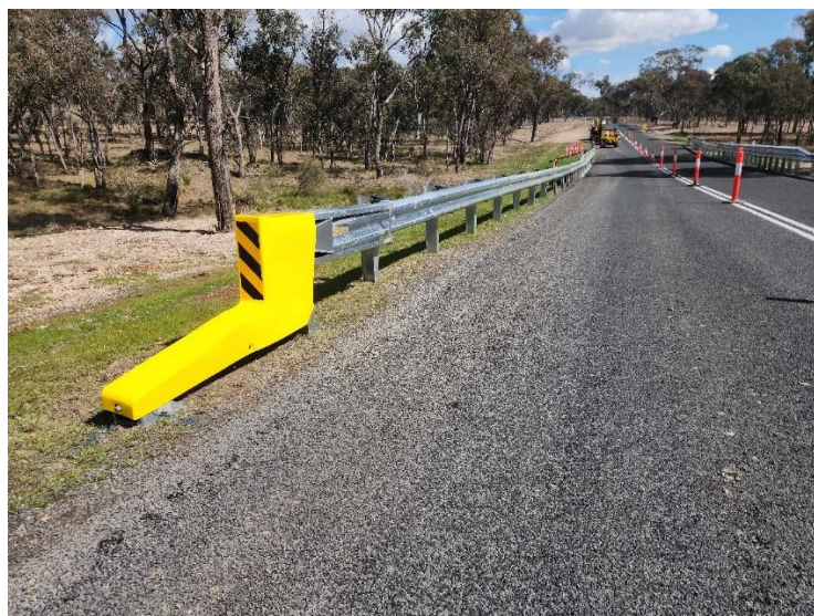
Image 2: Guard Rail installation
