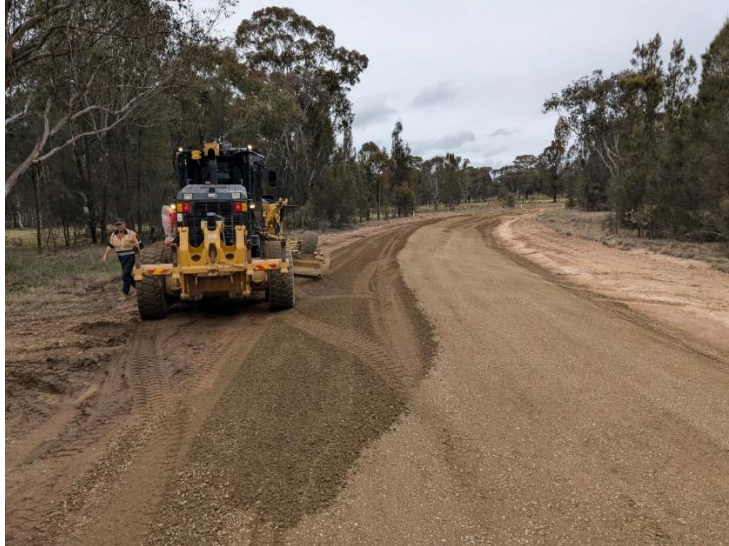
Image 1: Grader leveling Gravel
